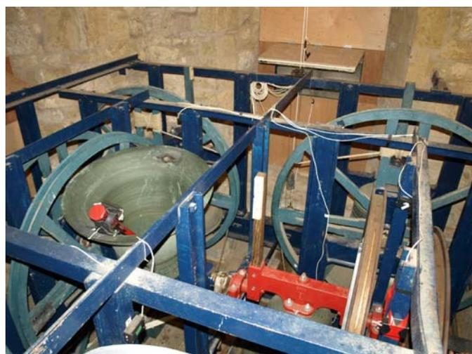
A view of the belfry: note wires from the sensors on the bells to the computer, the adjustable sound control, and the 'quickfit' car tyre bell muffle.
