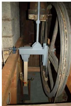
The dumb bell: note the old clock weights acting as a bell, and the interesting bungee 'slider' gear.
